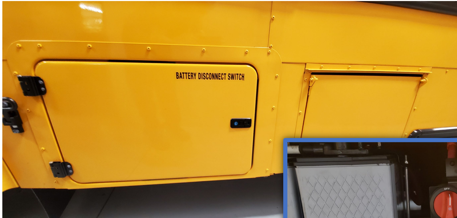
12V Battery Disconnect Switch
